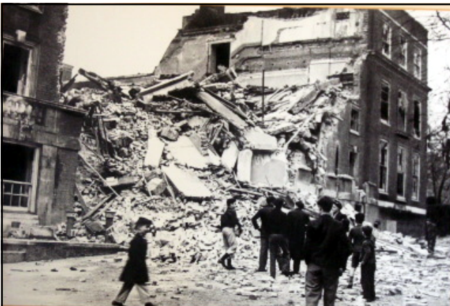
Bomb damage to KCHSS
